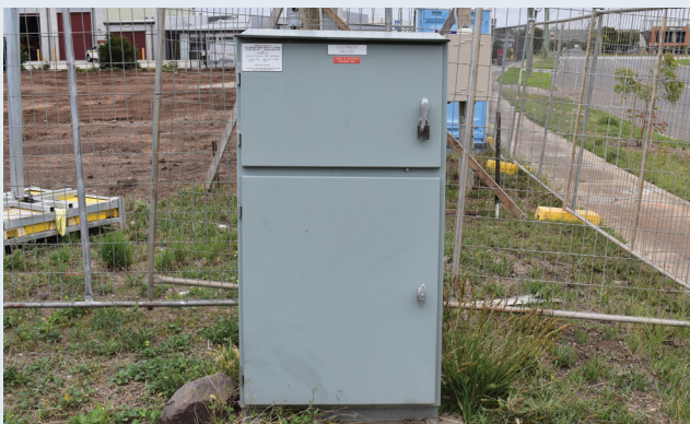
Figure 9: A customer switchboard and supply point for an electrical installation on private property.
