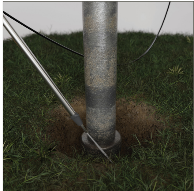
Figure 20: Two images showing the potholing technique.
