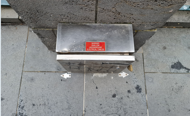
Figure 5: An electrical connection box providing warning that there are shallow underground electrical cables. Two arrow indicators showing the direction of the cables.
