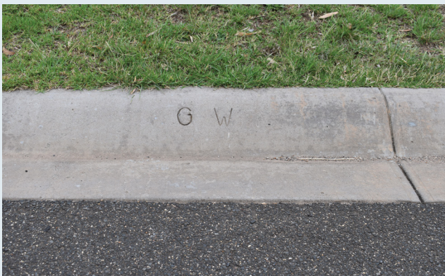
Figure 13: The markings "GW" (stands for Gas Water) on concrete guttering indicates gas and water assets beneath.
