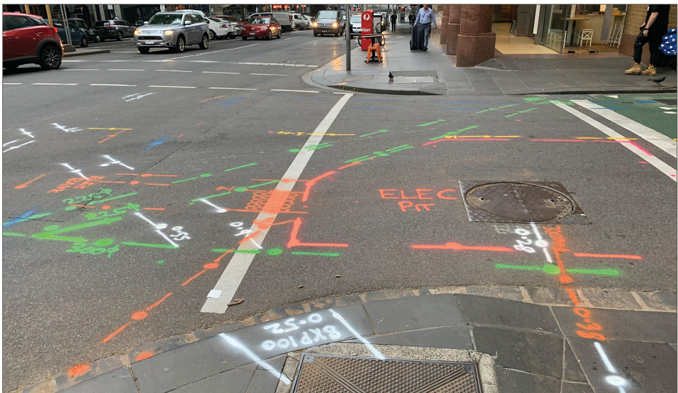
Figure 4: Example of paints used to mark underground services on roads and footpaths.
