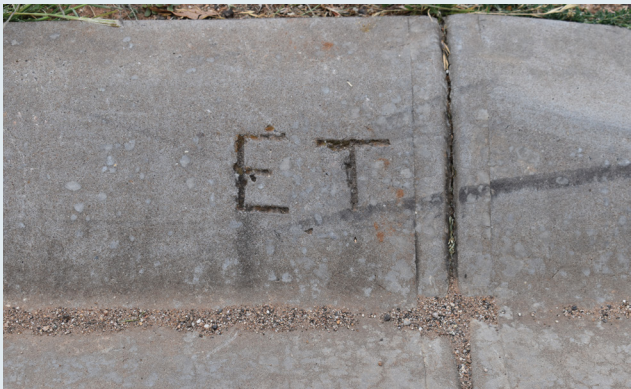
Figure 7: The markings "ET" (stands for Electrical Telecommunications) on concrete guttering indicates electricity and telecommunication assets beneath.
